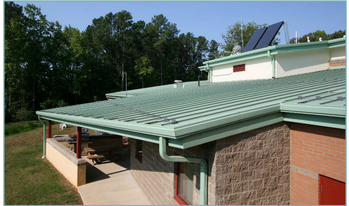
Solar roof panels and rain capture panels over patio
