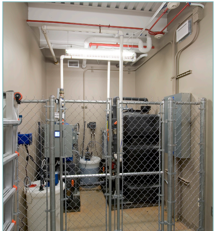
Water Reclamation System recycles rain that fall on the roof
